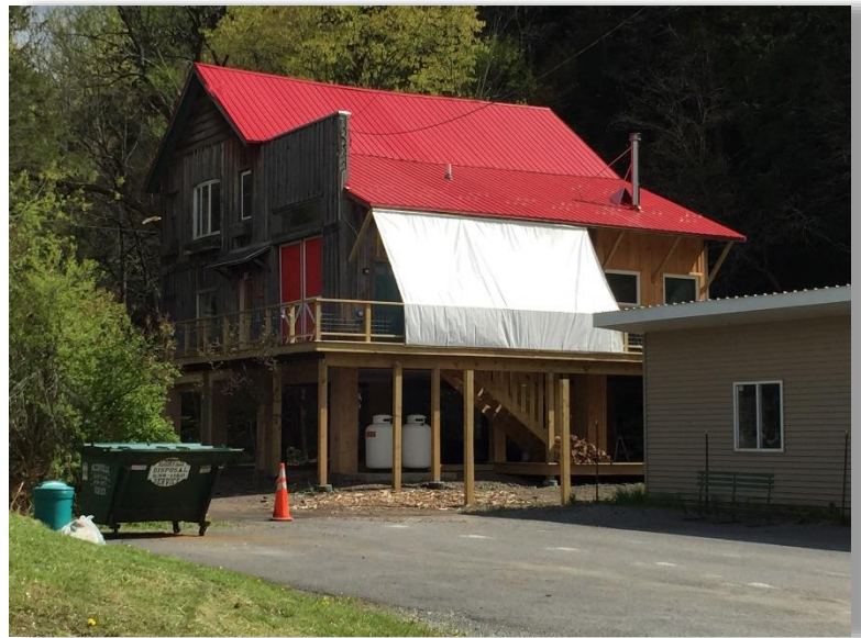
Figure 6-4 Example of an Elevated Structure
