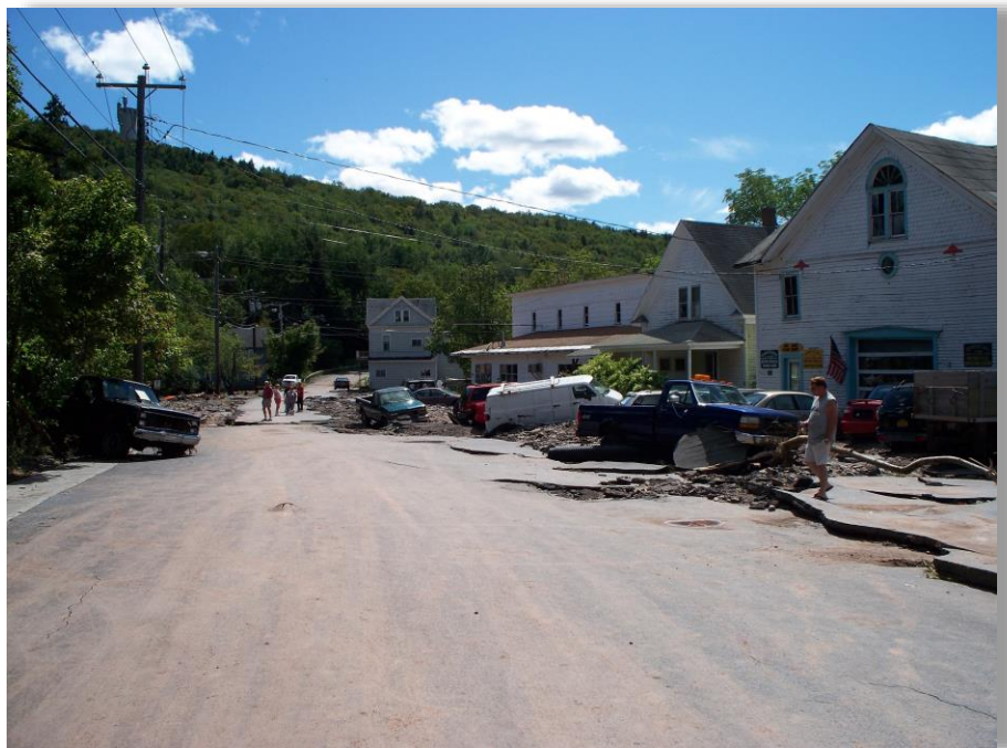
Figure 3-6 View of Railroad Avenue and Legg's Garage the day after the flood
